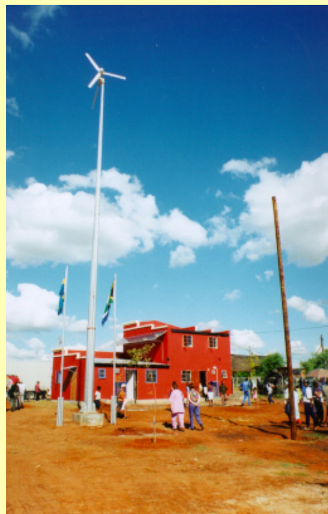
Figure: New 750 W wind turbine at the Moshoeshoe Eco-village supplying Green Power onto the grid
