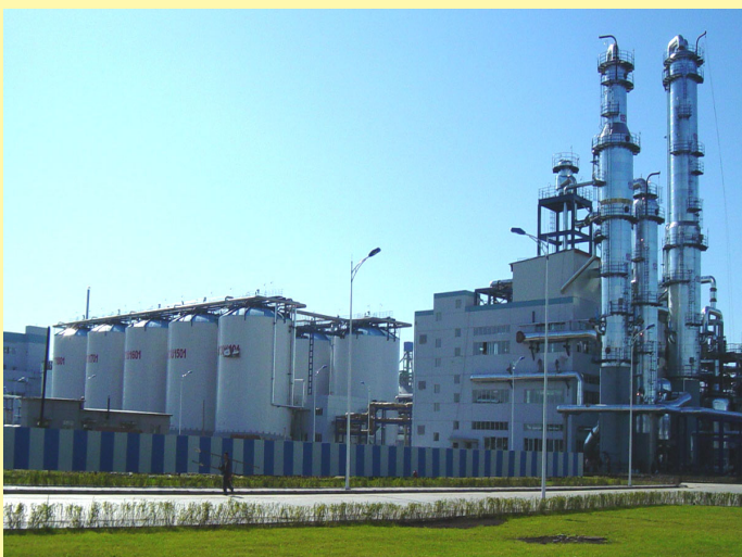
Figure: Fuel ethanol plant in Jilin, China
