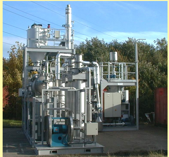
Figure 2: Fluid bed fast pyrolysis plant at Wellman, United Kingdom
