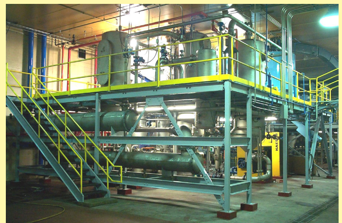
Figure 3: Ensyn Transported Bed fast pyrolysis plant at Red Arrow, USA
