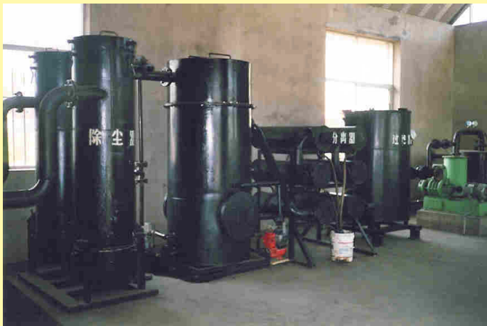
Figure: ENEA gasification plant in Beihai, China
