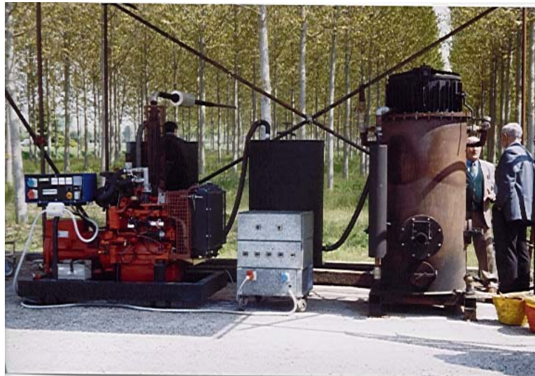
Fig. 1: Gasifier, gas filtration system and generator set
