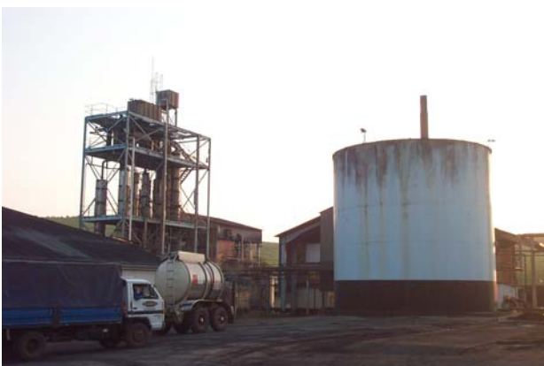
Pict. 24: Front: Molasse storage tank, Background: Distillation columns
