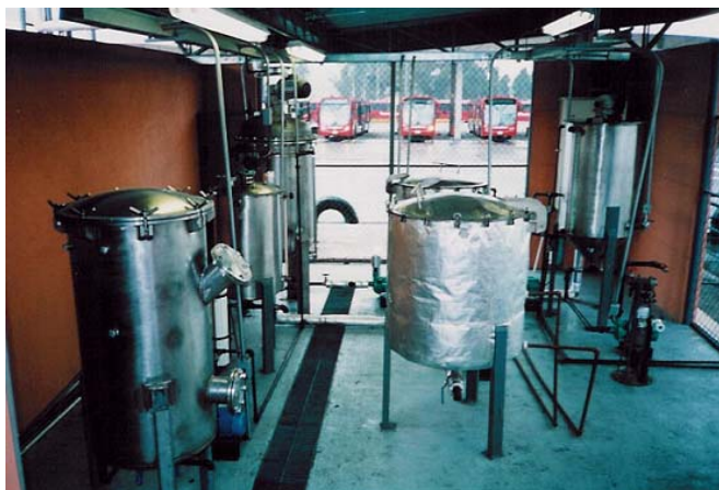
Figure 5: Bio-diesel pilot plant, Colombia (Source: CORPODIB)
