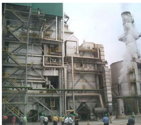
High pressure boilers at the Companhia Energética Santa Elisa
