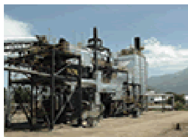
Termic plant, using sawdust and bark San Francisco de Moztazal, VI Region 25 ton/h steam generation
