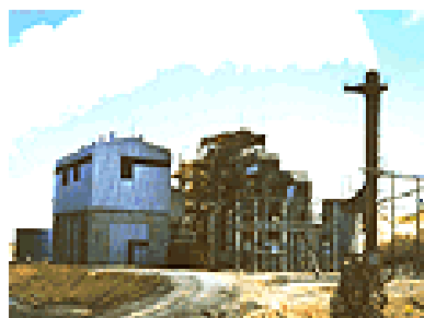
Termoelectric Plant using sawdust and bark from cellulose pulp plant Constitucion, VII Region 8,7 MW, 50 ton/h
