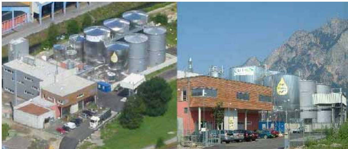
Biodiesel production facility in Arnoldstein, Austria
