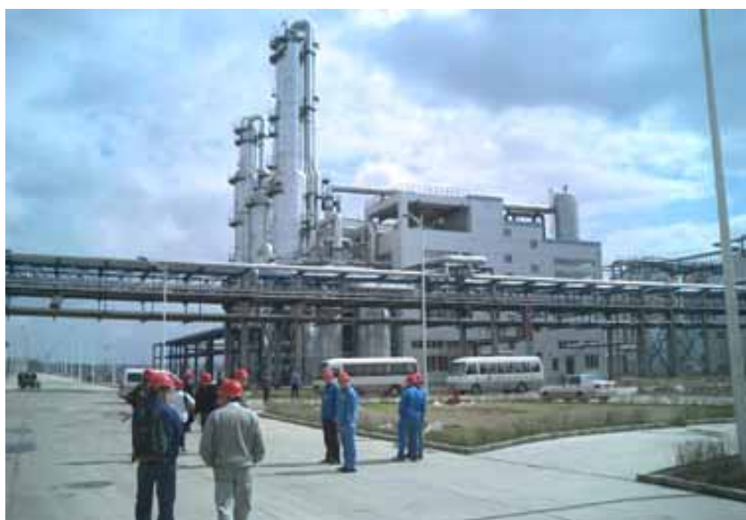
Bioethanol production facility in Jilin, P.R. China
