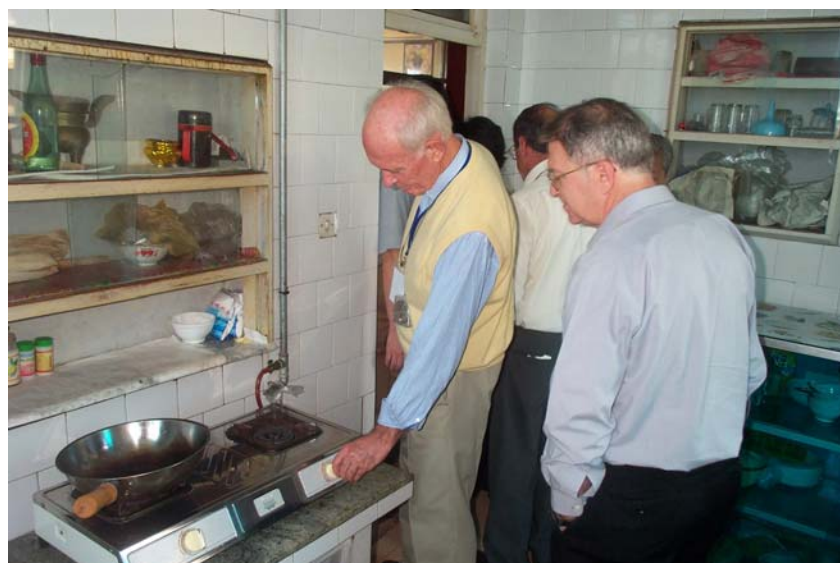
Fig. 7: Bio-gas burning cooking stove in operation
