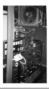
Design Shaft power system brushless AC electric generator
