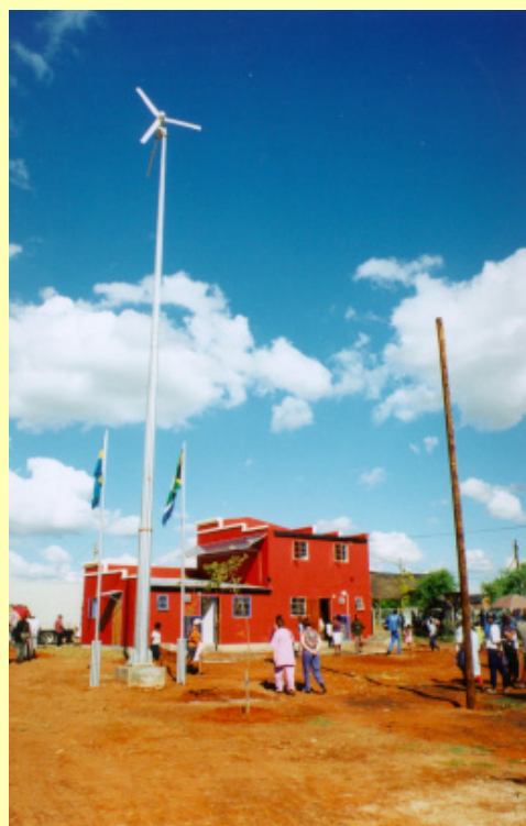
Figure: New 750 W wind turbine at the Mshoeshoe Eco-village supplying Green Power onto the grid
