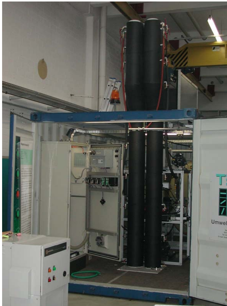
Figure 13: UASB-reactors at ISET e.V., Hanau/Germany
