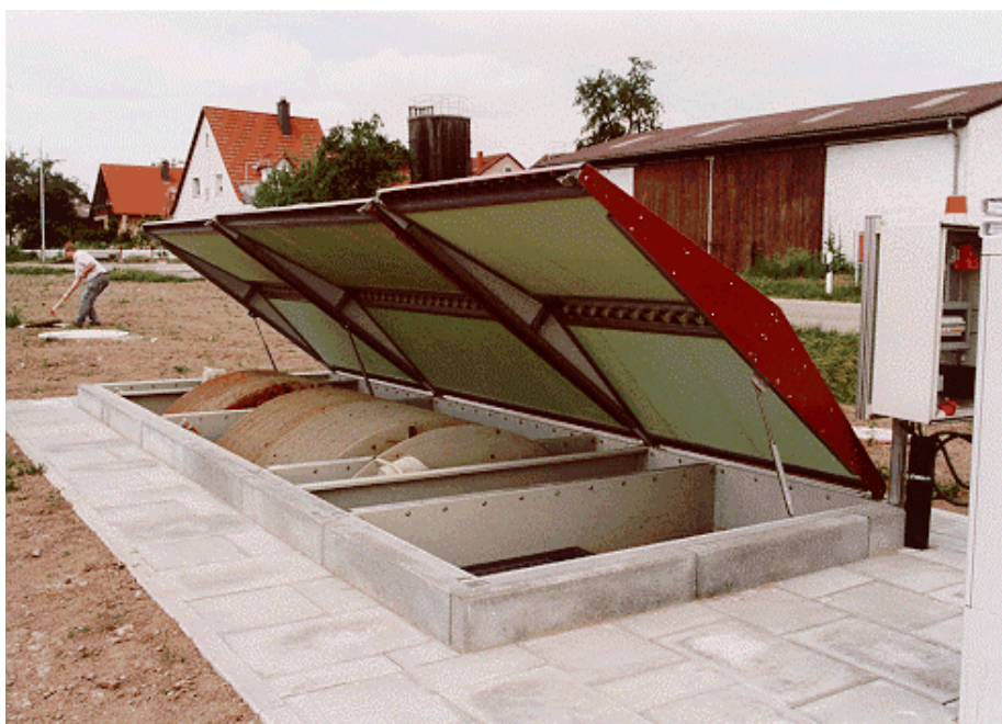
Figure 11: Rotating disc filters (Company: System S&P, Kirchberg/Germany)
