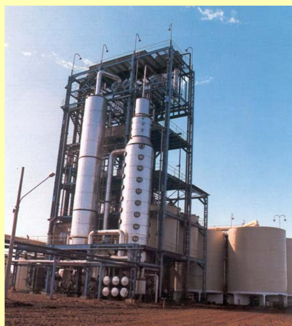
Distillation column from an ethanol production facility Source: Copersucar, Brazil
